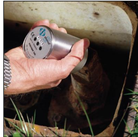
Figure 1 Phocus noise logger installation
