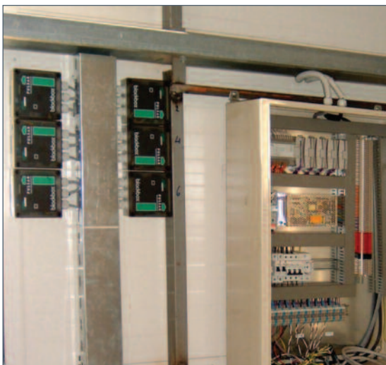
MINERAL OIL TANK LEVEL
